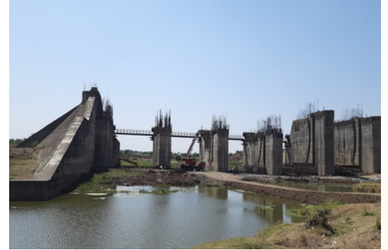
View of Pedhi Dam
