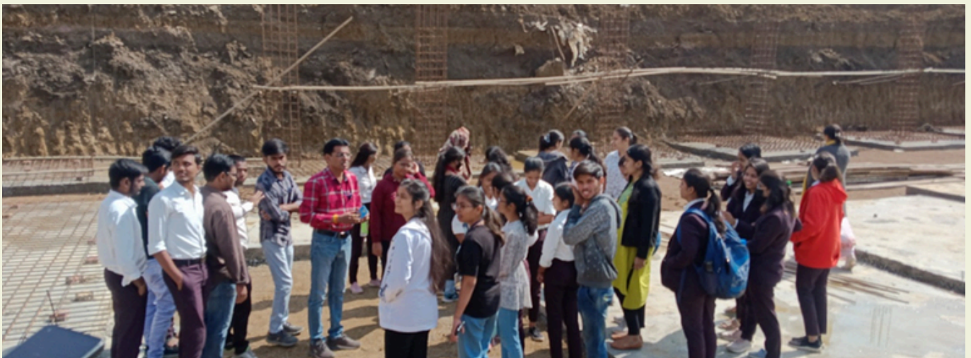
Images of site visit students observing the details of Column footings
