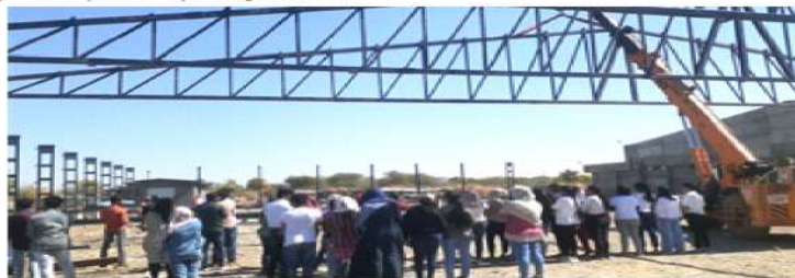
Lifting and Positioning of trusses at steel structure site.
